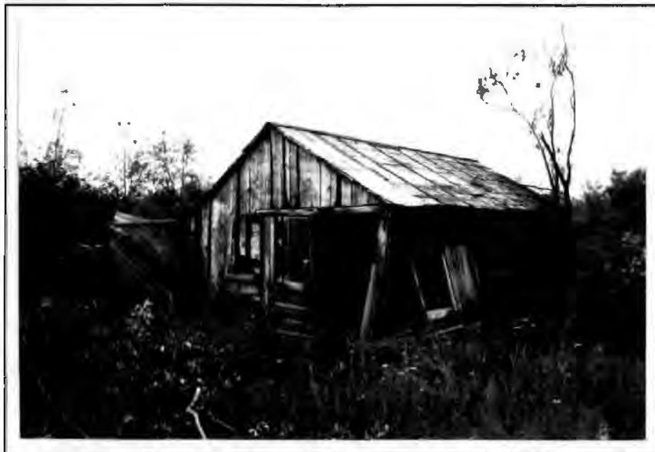
Figure 56. The Matheson Storage Building, 1993. The view is looking southwest.
